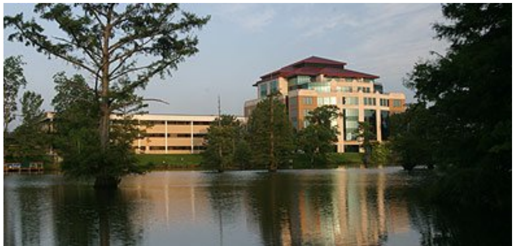
University of Louisiana Monroe Library on Bayou DeSiard
